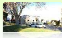
APLEX USA branch CA, USA
